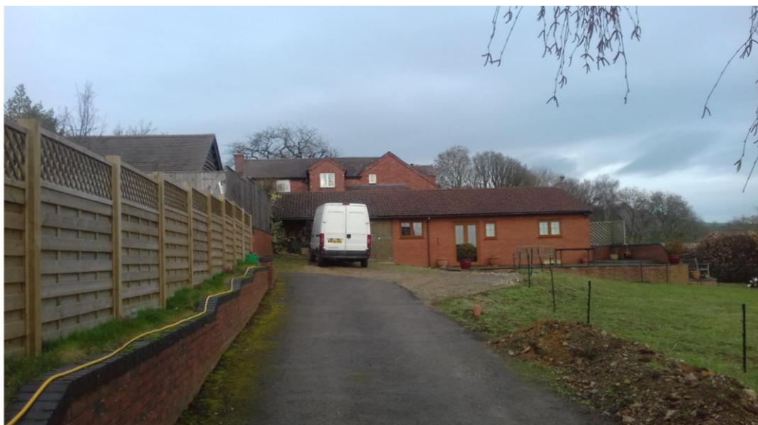
Figure 4 – Photograph of annex
